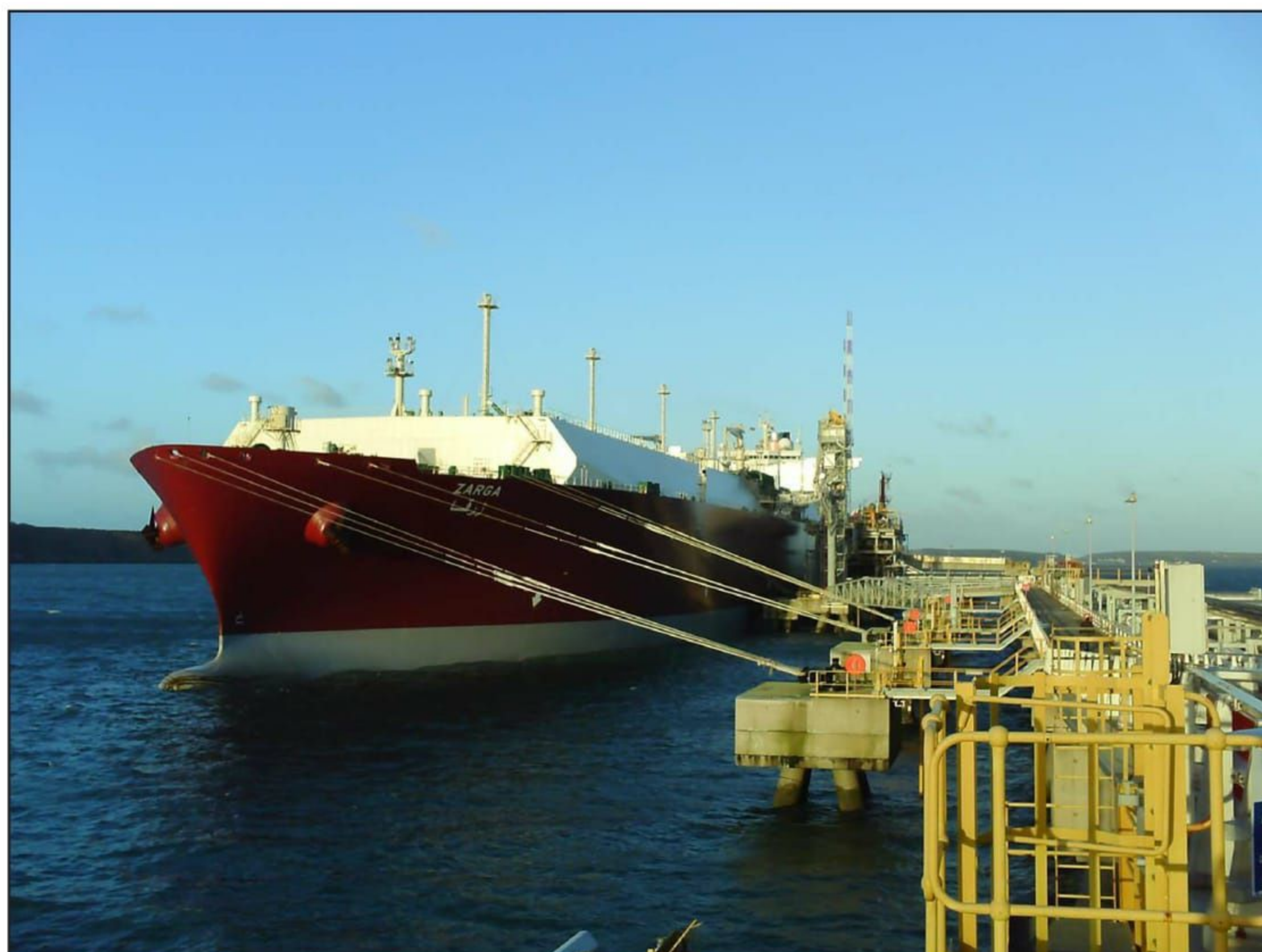
Figure 1: Zarga alongside South Hook LNG terminal
